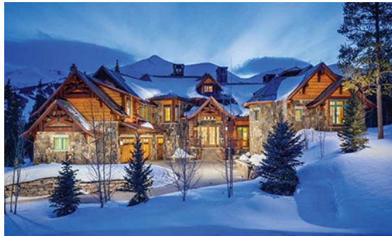
This 15,000-square-foot Colorado ski retreat features full Crest control of additional amenities such as the heated driveway, side melting system.
