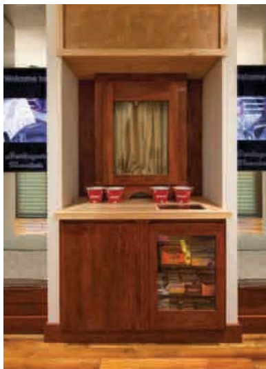
At the entrance to the theater, a snack counter with vertically mounted flat-panel displays on each side.
