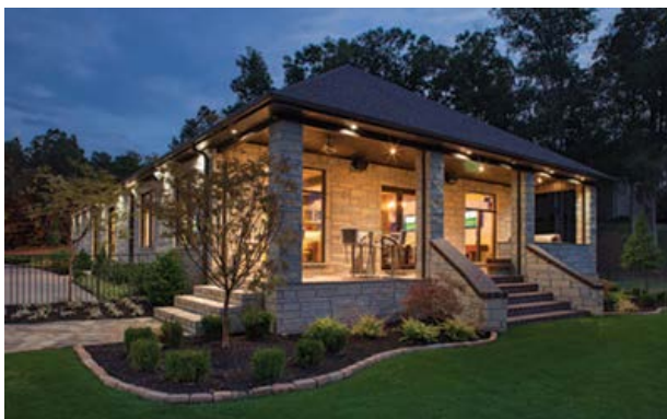
The man cave is a 4,000-square foot freestanding structure next door to Ryan Heringer's house. The patios feature outdoor speakers and TV and motorized mosquito screens integrated into the Crestron system.
